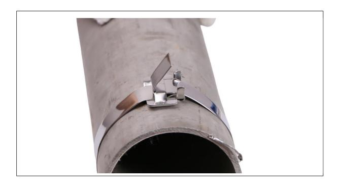
(7) Knock the stainless steel belt into the packing buckle with a hammer, and then use a hammer to hit the ears of the packing buckle to both sides of the stainless steel belt to fix the packing buckle.
